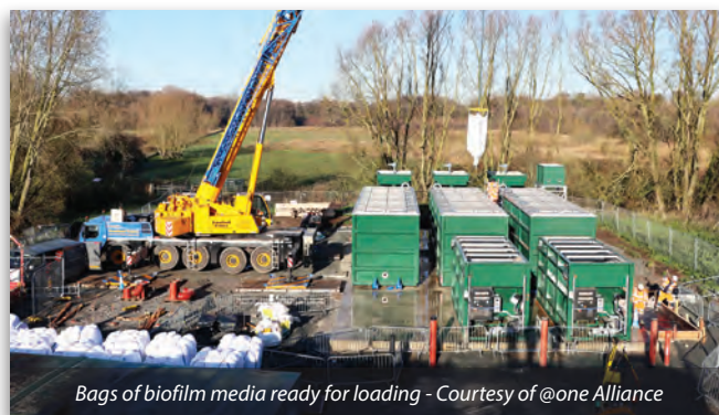
Crane lift for MBBR media - Courtesy of @one Alliance
