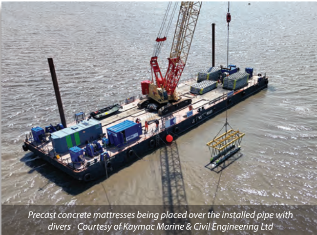
Concrete mattresses being placed over submerged pipe during night shift Courtesy of Kaymac Marine & Civil Engineering Ltd
