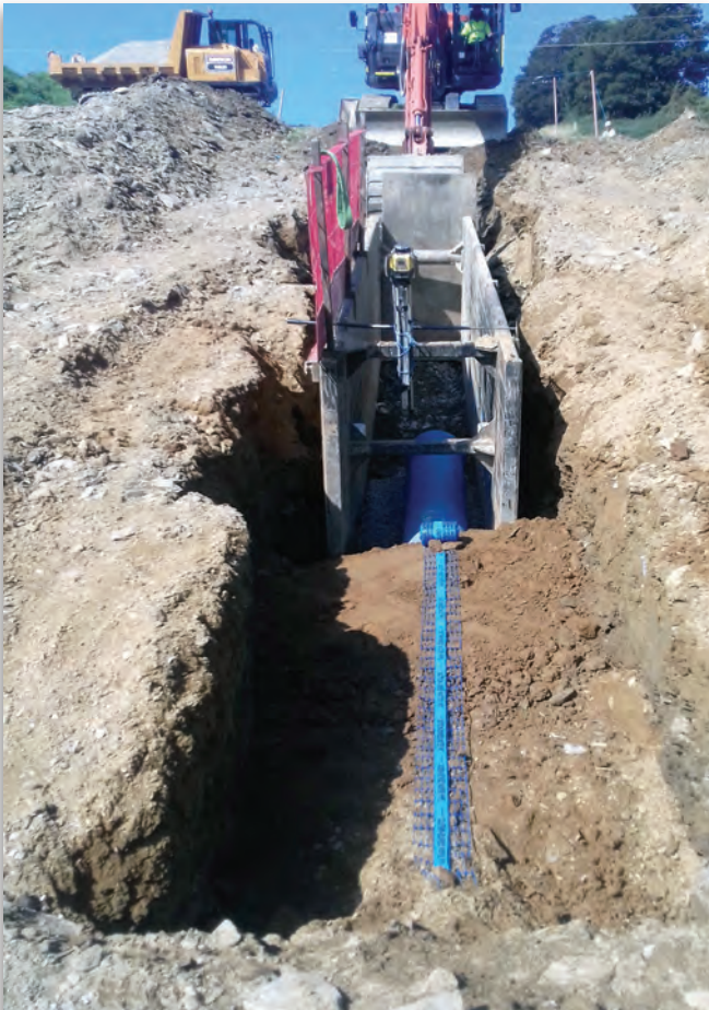
Mains laying operations - Courtesy of DAWSON-WAM & NI Water
