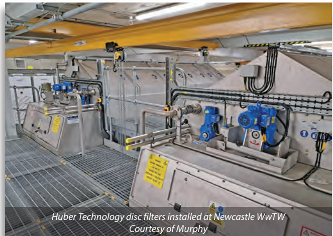
Tertiary filters inlet control valves - Courtesy of Murphy
