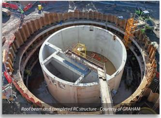
large access covers for the three submersible pumps and two mixer pumps. The roof deck consisted of 22 precast slabs, which were cast off site due to insufficient space on site. The largest slab weight was 14 tonnes.
