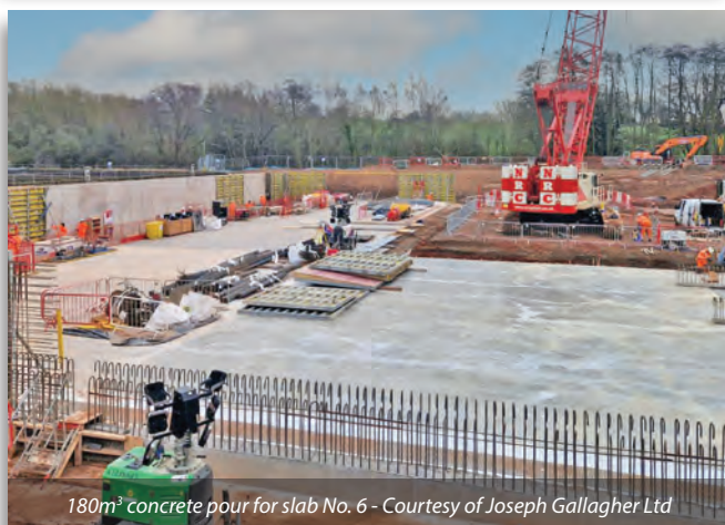
Slab construction and start of wall shuttering placement - Courtesy of Kier
