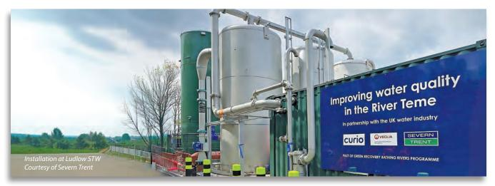
The modular design of the ozone plants, pre-assembled in shipping containers, enabled rapid deployment and minimised disruption to existing site operations. This approach not only reduced construction time and carbon footprint but also provided a scalable model for future installations. The closed-loop ozone systems, equipped with real-time monitoring and automated destructors, ensures safe operation.
