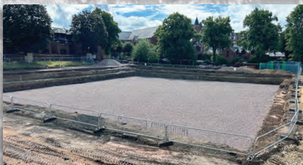
Construction of the 2 megalitre attenuation tank - Courtesy of Forkers Ltd
