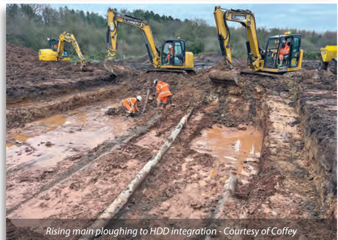
Rising main ploughing to HDD integration - Courtesy of Coffey
