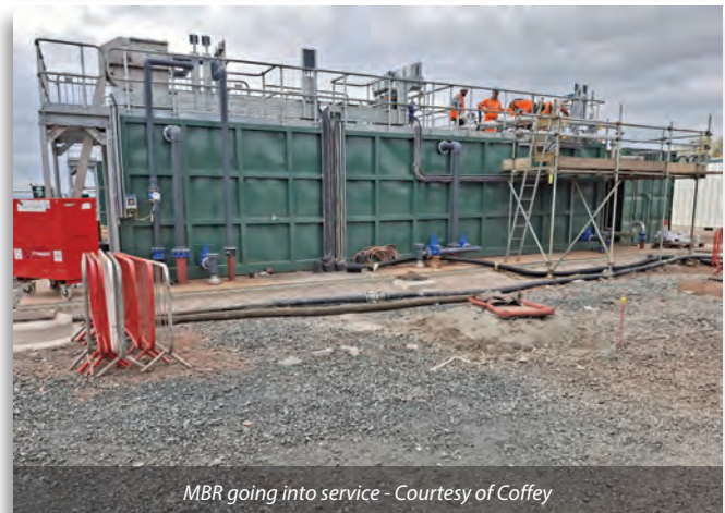
MBR Stream 1 fit-out - Courtesy of Coffey
