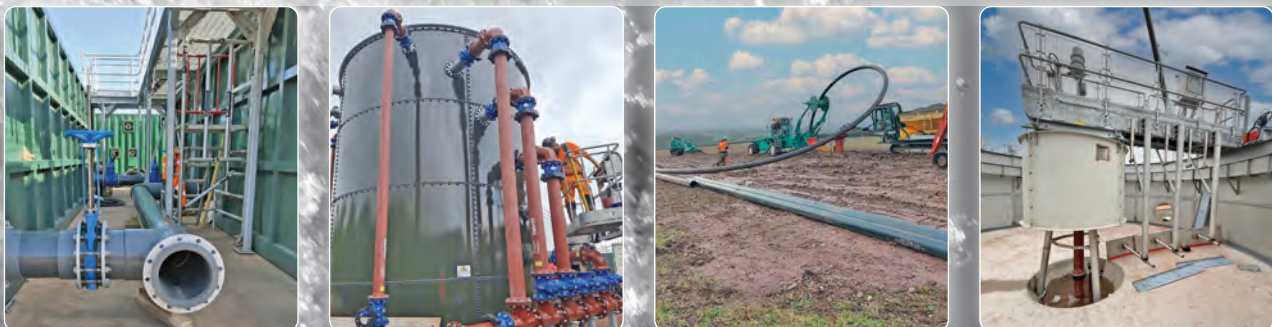
(left to right) MBR interconnecting pipework, sludge tank, pipe ploughing operation, and PST bridge scraper - Courtesy of Coffey
