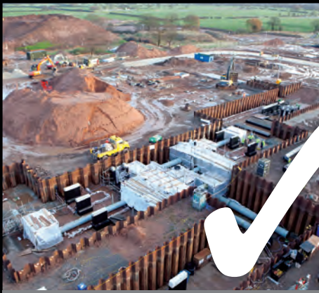
TEMPORARY SHEET PILING
