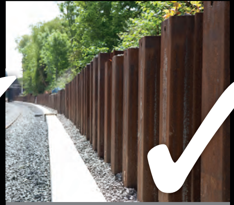
PERMANENT RETAINING WALLS
