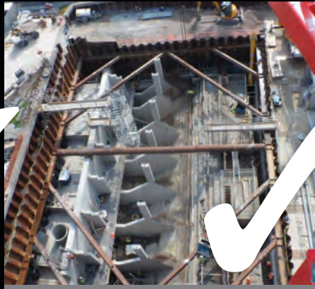
TEMPORARY BRACING
