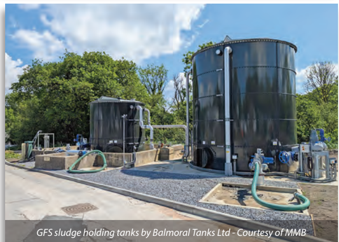
Two additional COUFs were incorporated to accommodate increase in flows to be treated - Courtesy of MMB
