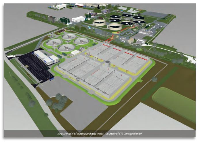
**Sequencing Batch Reactors (SBR):** Eight new SBR basins are required, each 30m wide x 60m long 7m high, with a capacity of more than  $12,500m^3$  each.
