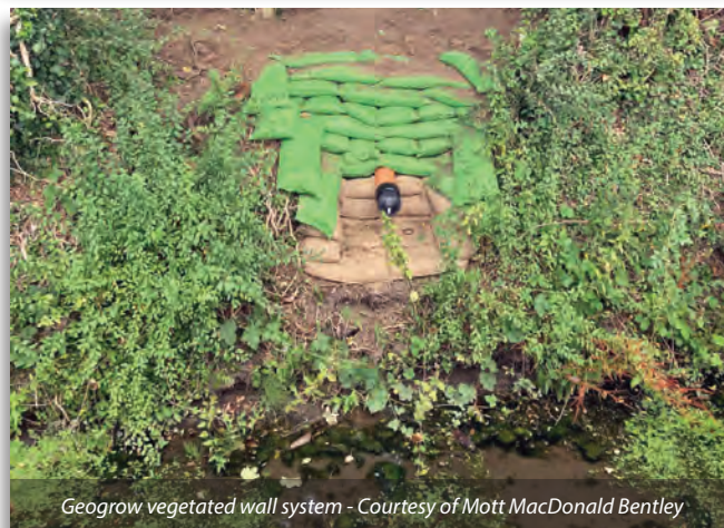
Installation of the vegetated wall system Courtesy of Mott MacDonald Bentley
