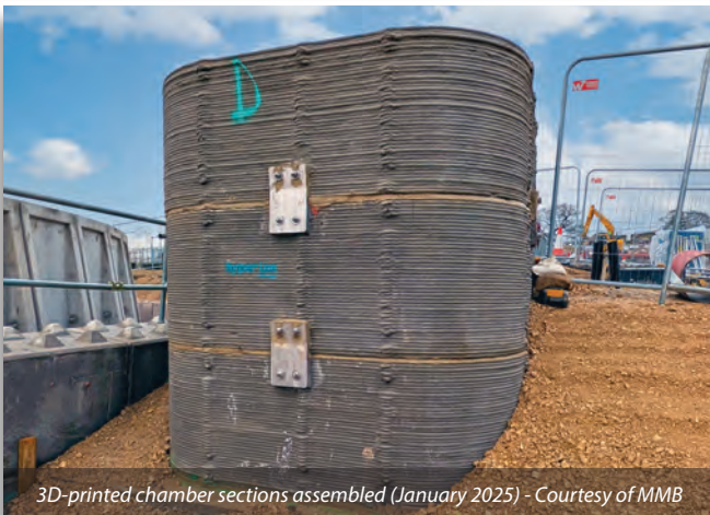
3D-printed chamber sections awaiting installation (September 2024) Courtesy of MMB
