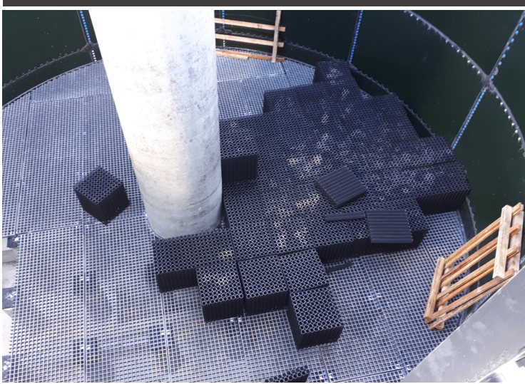
Sandbach Project NTF bio-tower under construction - The bottom layer of BIO-BLOK being installed inside a new Sandbach Works NTF bio-tower onto the GRP support deck mounted on concrete piers.
