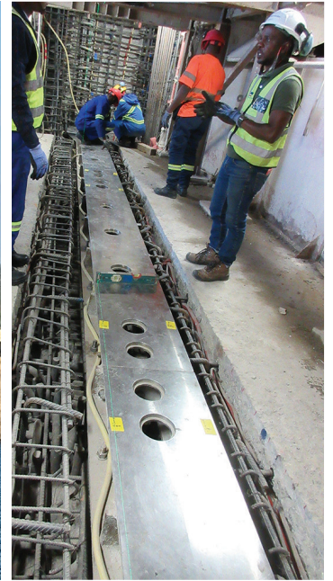
KGAL design sill being aligned in Sluice 3
