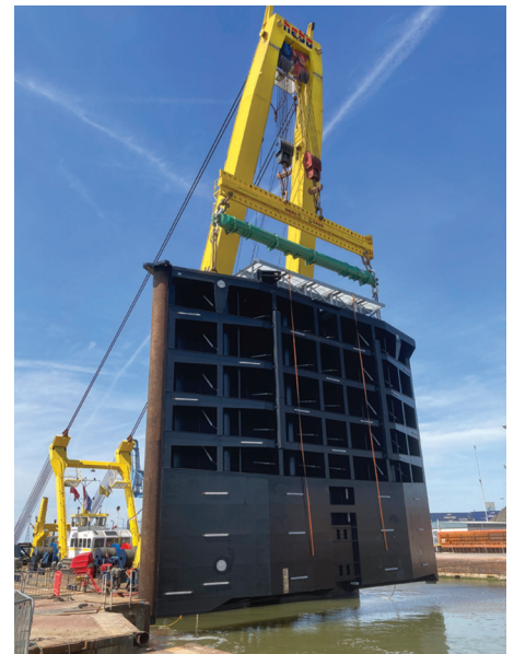
Current radial gate installation
