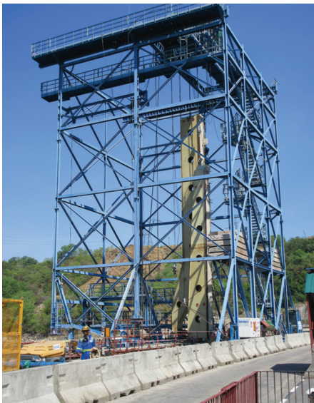
Needle C1 of Cofferdam 1 being transferred between Sluice 6 and 5
