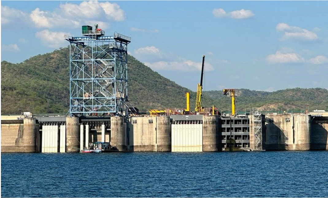
View from the upstream side with Sluice 6 on the left, showing the transfer of Cofferdam 1 between Sluices 6 and 5, Cofferdam 2 in Sluice 3 and the stoplogs in Sluice 2
