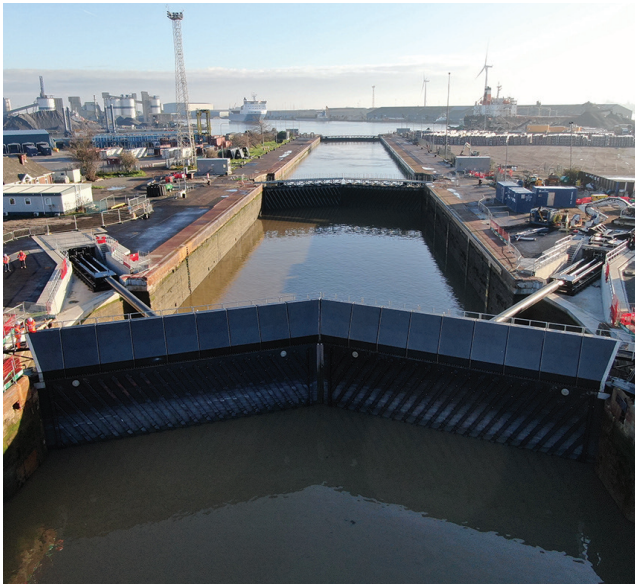
New lock gates and associated infrastructure at Tilbury
