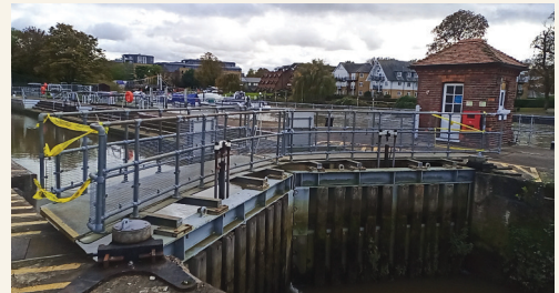
View looking upstream at the existing tailgates and Launch Lock
