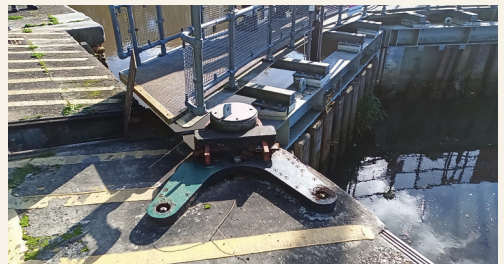
View of existing gate, top anchor and cylinder pit
