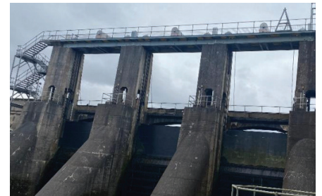
The spillway gates at Cliff Dam
