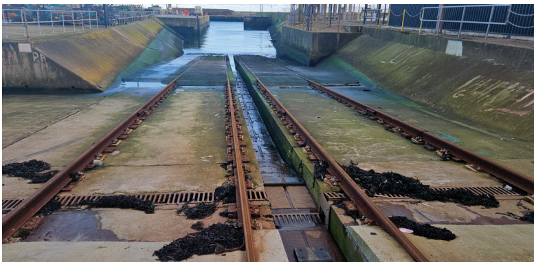
Site photo showing where the new cradle will be positioned
