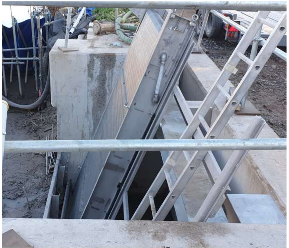
Both screens were in position within a few hours. Most of that time was due to crane availability: The screens slide into place on the pivoting frames and are then leaned back onto the I-beam that spans the chamber.
