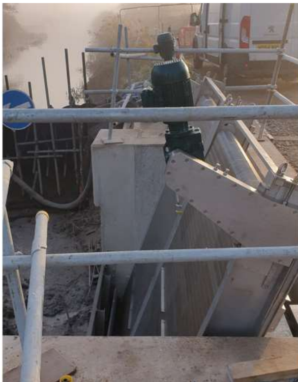
Both screens were in position within a few hours. Most of that time was due to crane availability: The screens slide into place on the pivoting frames and are then leaned back onto the I-beam that spans the chamber.
