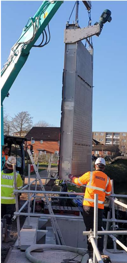
First screen being lifted into position.
