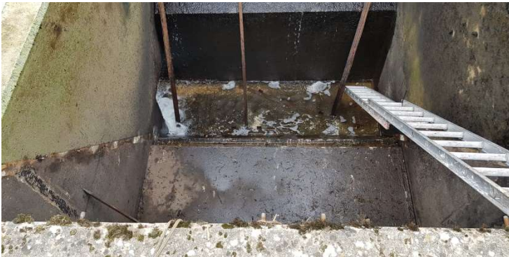
Intake chamber with the old static screens removed and waiting for the new GoFlo screen Baseplates to be fitted.
