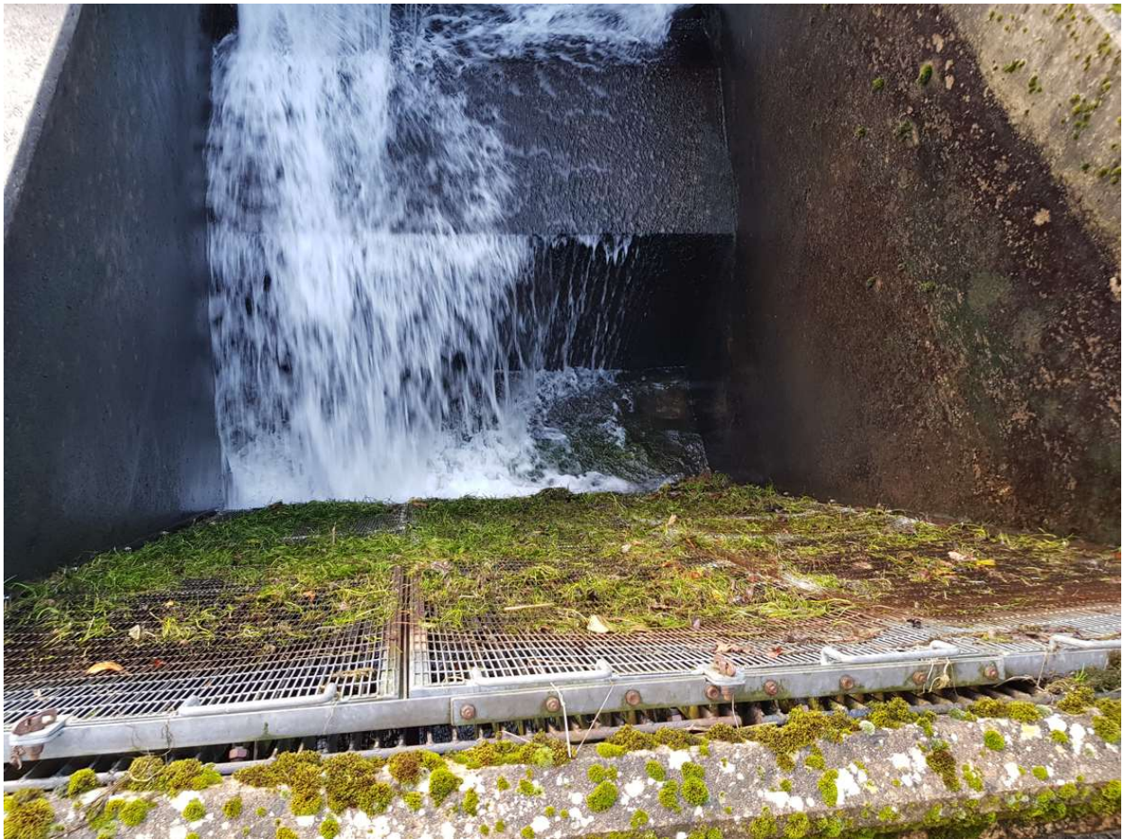
Smolt screens installed on top of the bar screen.
