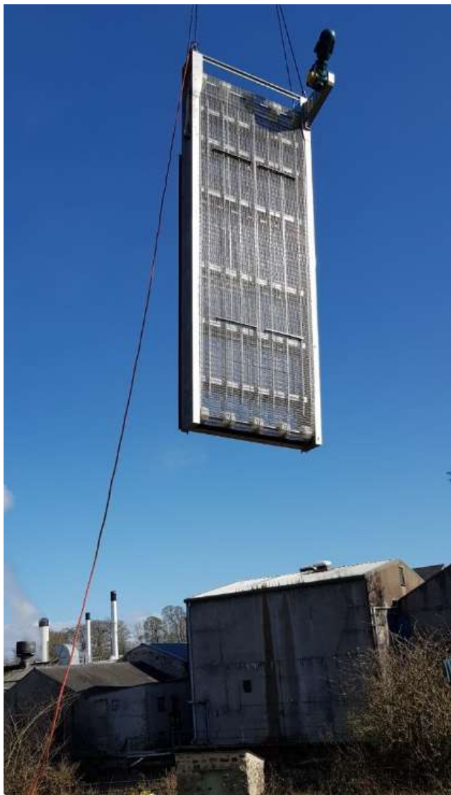
GoFlo screen no.1 being lifted over the trees to the intake.
