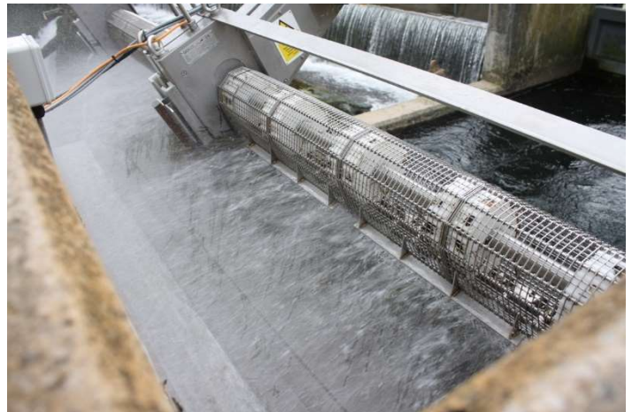
Screen washing: Both screen's spray bars operate simultaneously for the duration the screens cleaning cycle.
