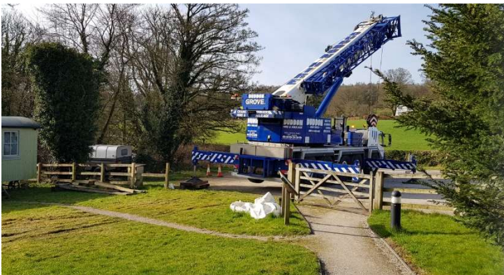
A 100-Tonne crane had to be employed to lift the new equipment into position; not because the equipment was particularly heavy, but because a long reach was required (30 m) to bridge the gap between the channel and the solid ground the crane could stand on.
