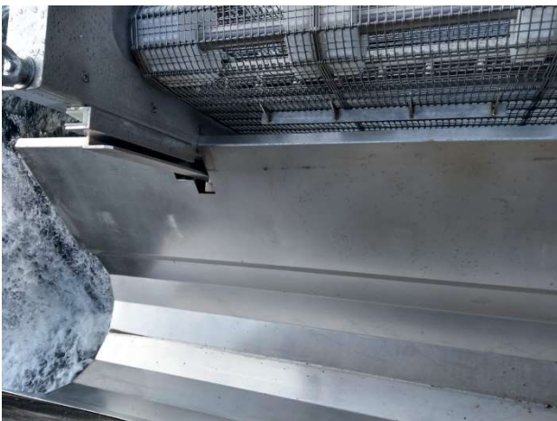
Debris trough – discharge end spills into the river downstream of the weir.
