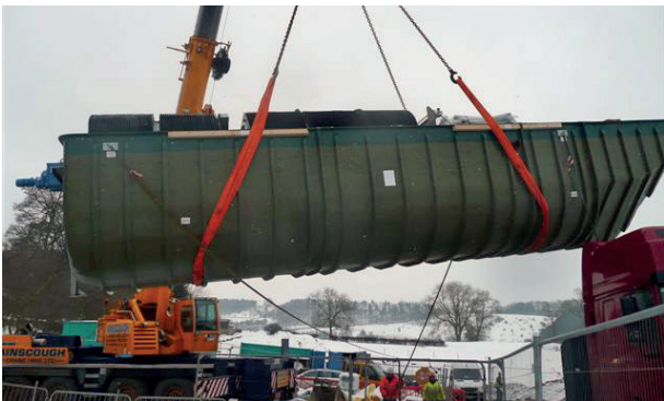
NuDisc® 5000 - being off-loaded onto concrete slab
