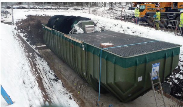
NuDisc® 5000 – successfully delivered and off-loaded at site in Derbyshire
