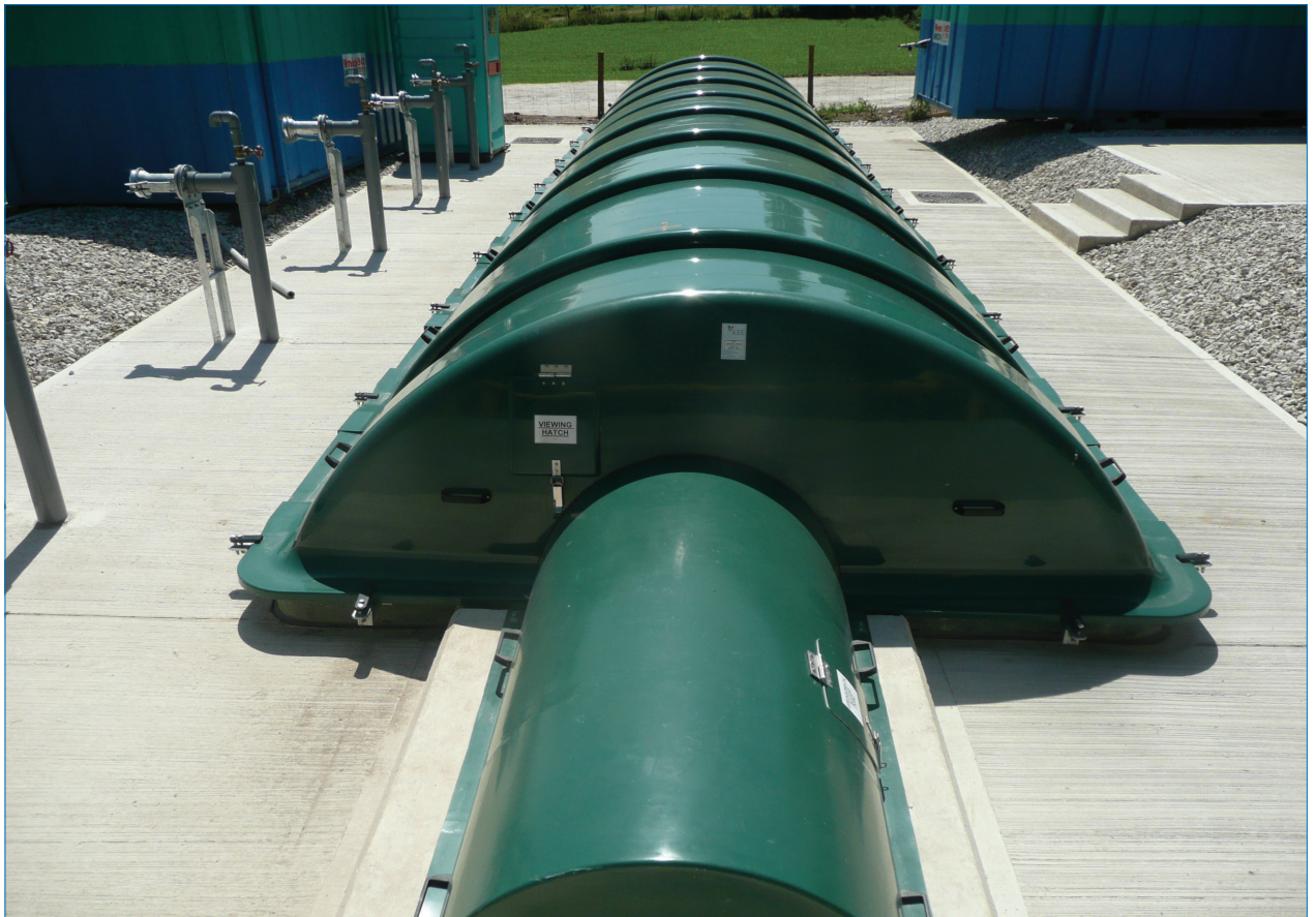
KEE NuDisc® 5000 ready for receiving flows (showing remote de-sludging ports)
