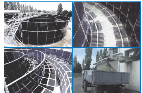
Multi-stage Submerged Aerated Filter Plant. Preliminary treatment includes screening.
