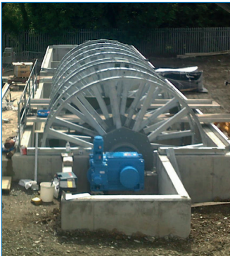
Keady WWT Works, Large diameter RBCs under construction
