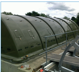
Keady WWT Works, Large diameter RBCs under construction
