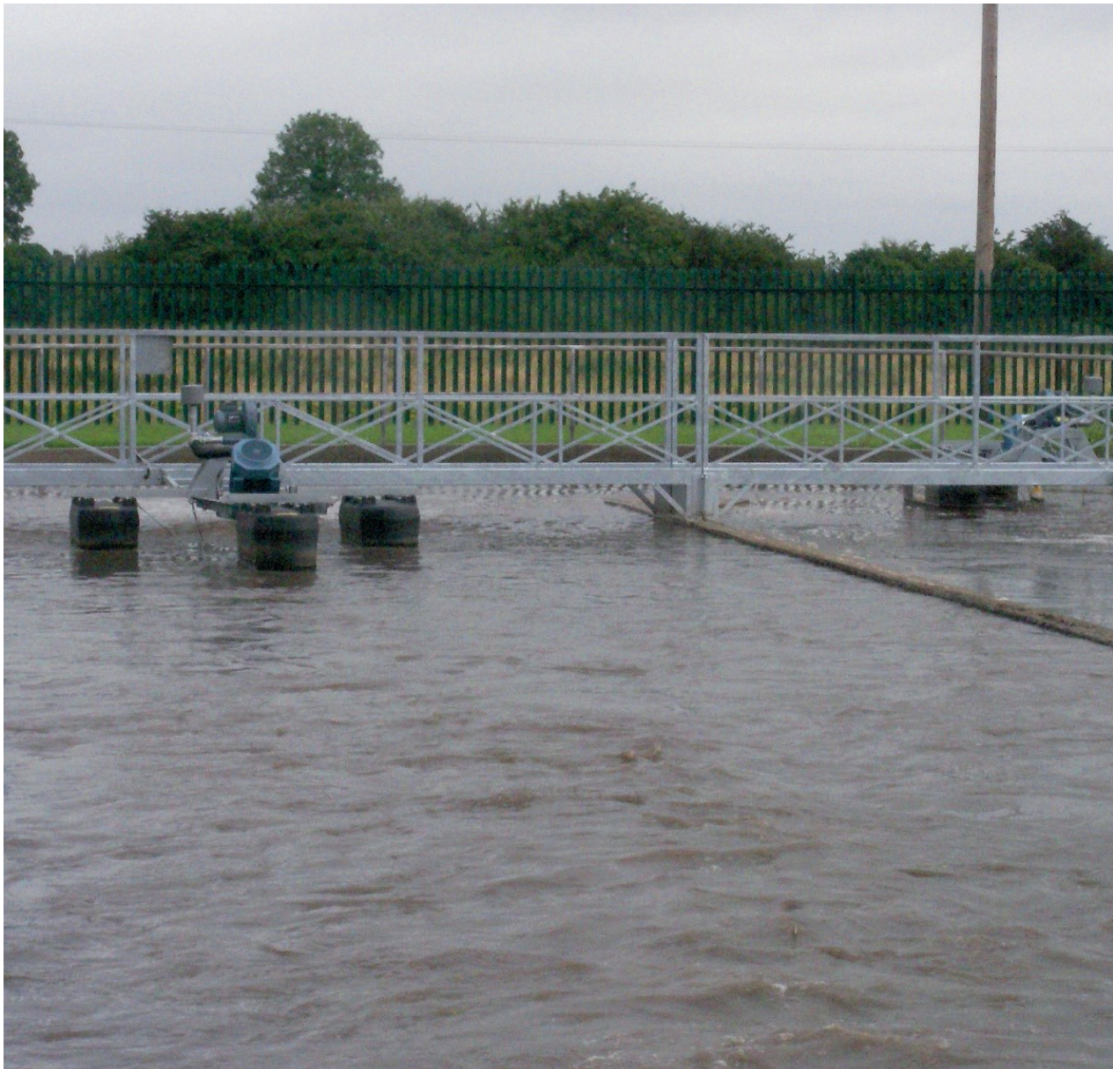
3.7kW Tritons® on a tri-pontoon float in position and fastened to the access gantry. The Triton® can be bridge or side-wall mounted.
